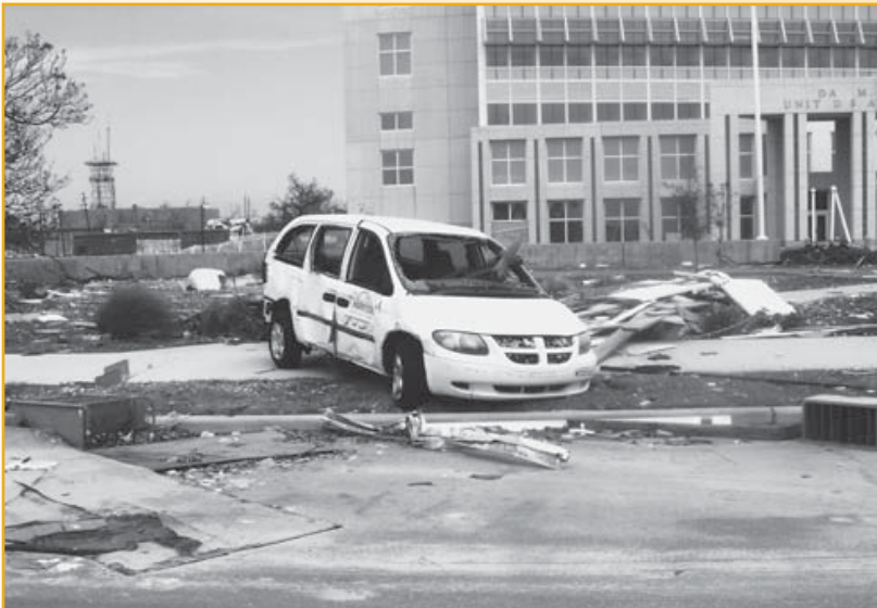
Federal buildings and U.S. courthouses damaged by Hurricanes Katrina and Rita will be cleaned up and repaired with supplemental funding provided to GSA in FY 2006.
